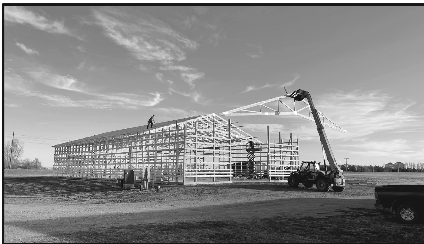
Rafters being placed at the Oakes Irrigation Research Site.
