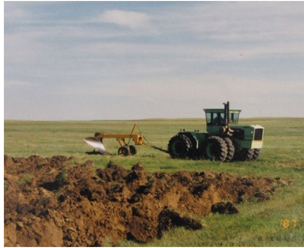
Figure 15. A plow used to mix amendments to a depth of about 4 feet. (NDSU photo)
