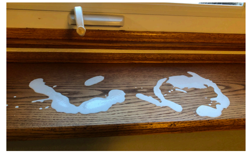
Fig. 4 In a second attempt to remove the stains, a paste of water and Bar Keepers Friend was spread over the stains and left to dry.
