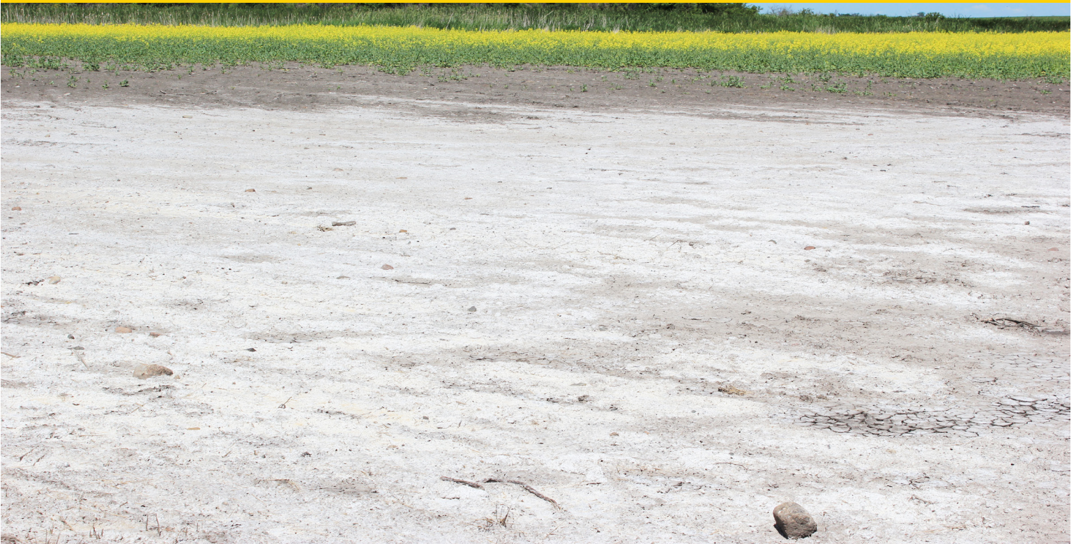
Figure 1. A typical saline spot along state Highway 17 East, N.D.
